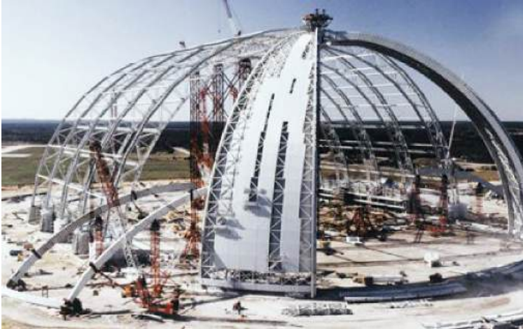
CargoLifter hangar under construction. Sources: (L) Beyond Plan B , (Below) Screenshot, Nils F time lapse video (May 2000 image).
