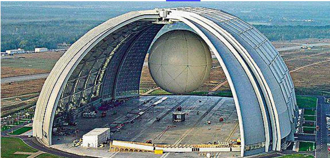
The completed CargoLifter hangar with the CL75 AC transport balloon inside.
