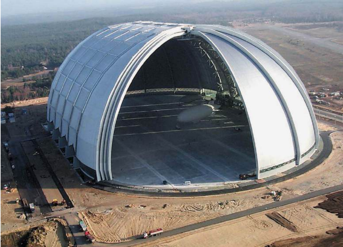
The completed CargoLifter hangar with Skyship 600B training airship inside.
