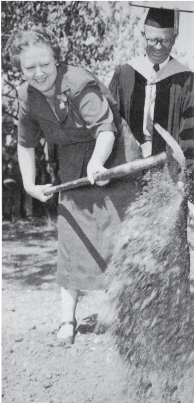
Mrs. Score turns a shovel of dirt for the beginning of work on the chapel in 1949 as I. J. McCook looks on. From the 1950 Southwestern .
